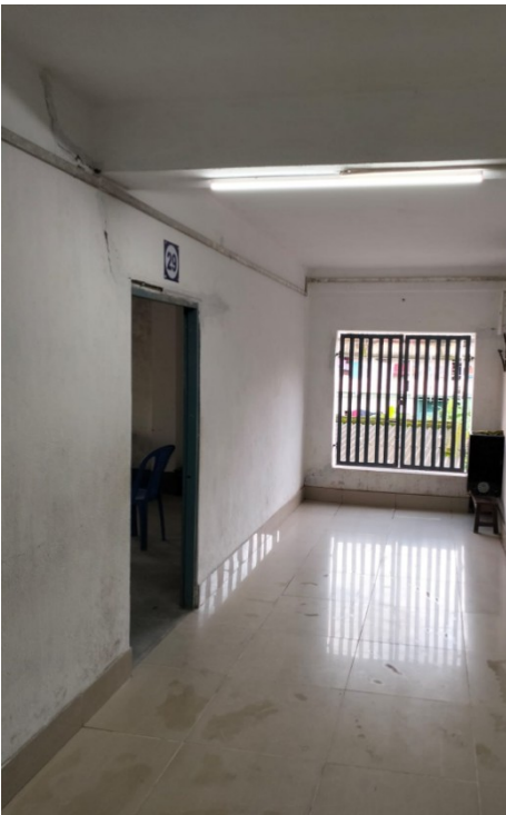
The entrance to the Balcony
