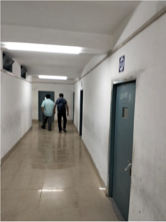
The passage besides the classrooms
