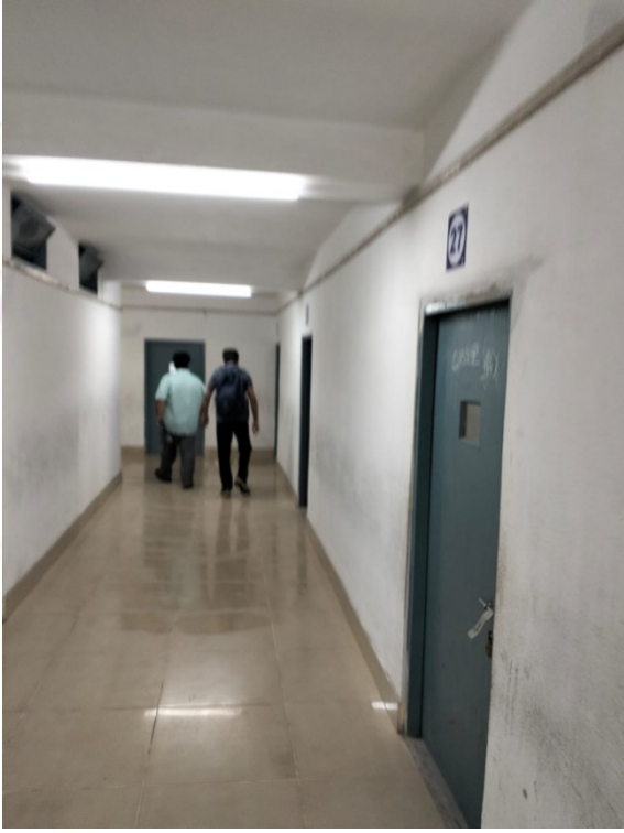
The passage besides the classrooms
