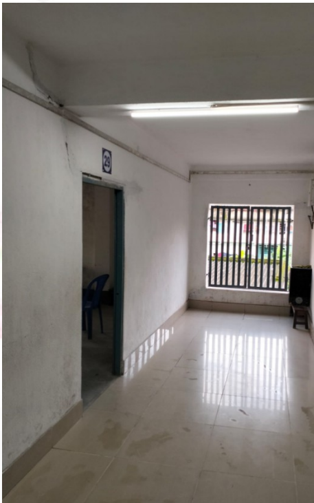
The entrance to the Balcony
