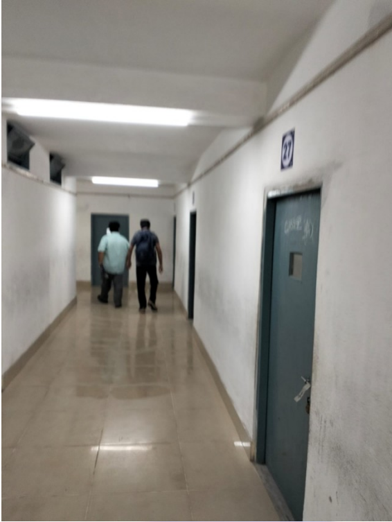
The passage besides the classrooms
