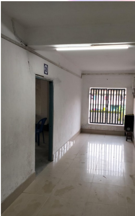
The entrance to the Balcony
